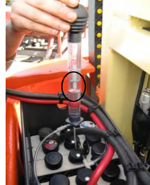
Figure 8-4. Measuring Electrolyte Specific Gravity
